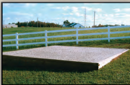
Framed-In Limestone Base
