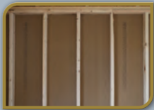
Wall studs 16" on center
