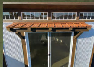
Awning with copper roof for dbl door & single door
