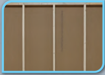
Wall studs 24" on center
