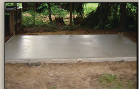
Reinforced Concrete Slab
